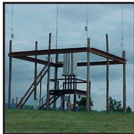
Launch platform & conductor masts
